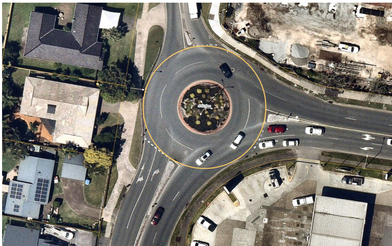
Figure 11: Darlington Drive / Leisure Drive Roundabout (Source: Nearmap)
